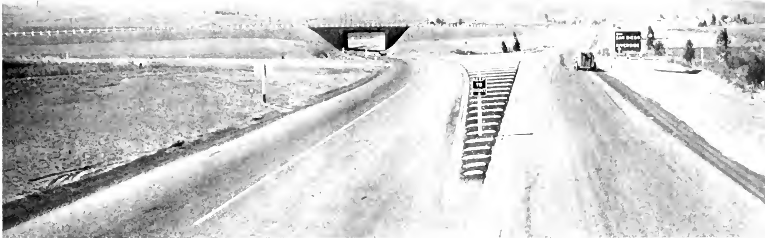
Top—View west. Pepper trees previously bordered old two-lane road. One row now in dividing strip. Center—Dual roadway sections each paved 23 feet in width. Dividing strip is 30 feet wide between near edges of pavement. Bottom—View west. Island between traffic channels constructed of bars made of plant-mixed surfacing and painted white. Grade separation structure in center.
